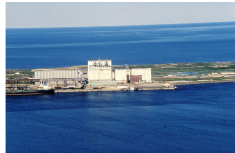
Grain Elevators Churchill, Manitoba
